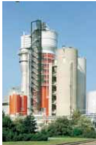
Flue gas desulphurization at the Preussen Elektra power plant, Wilhelmshaven, Germany.
