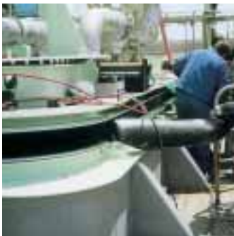
▲ The "Piper" feed unit (ELF Enterprises) equipped with Fluastal® fabric expansion joints on the gas turbine exhaust ducts.
