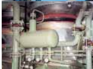
Ventilators (Howden Variax) in the St. Gotthard tunnel, Switzerland, with KE-Burgmann expansion joints.
