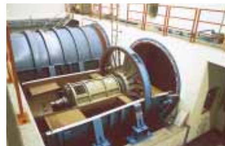
Ventilators (Howden Variax) in the St. Gotthard tunnel, Switzerland, with KE-Burgmann expansion joints.
