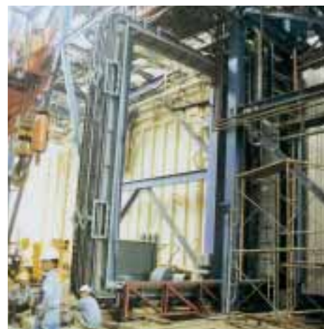
▲ Combined Cycle Power Plant 'Tanjung Priok', Jakarta, Indonesia. Fluastal® multilayer expansion joints installed after the turbine (ABB 13E) and on the boiler (double expansion joints with scissor control guides).
